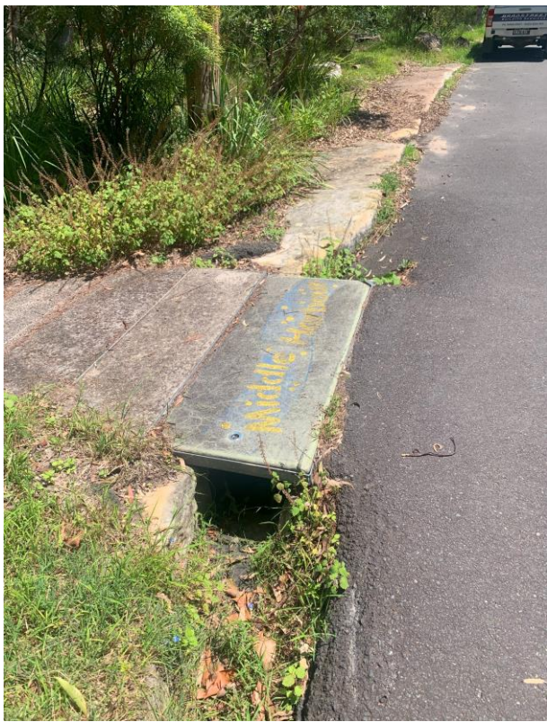
Figure 2: Later concrete lid placed over the culvert on the southern side of The Rampart.
