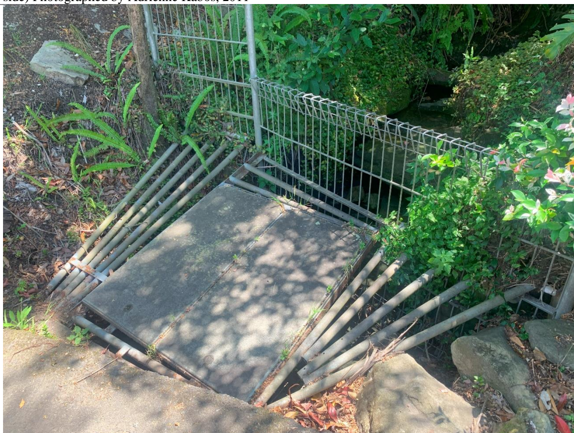
Figure 3: Concrete cover and metal fencing around the northern inlet.
