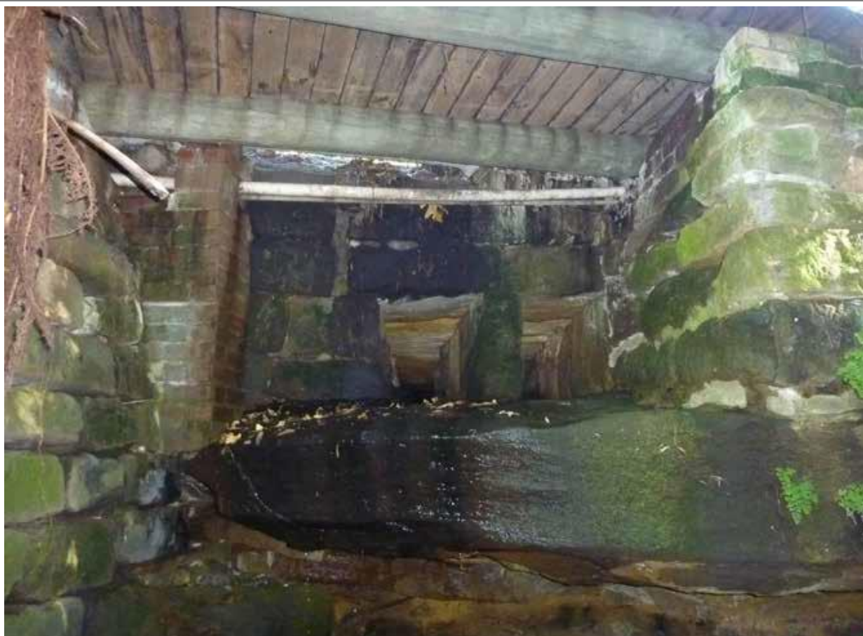
Figure 2: The flat roofed bridge showing the twin channels and abutments on the Retreat Reserve side (southern side) Photographed by Adrienne Kabos, 2011
